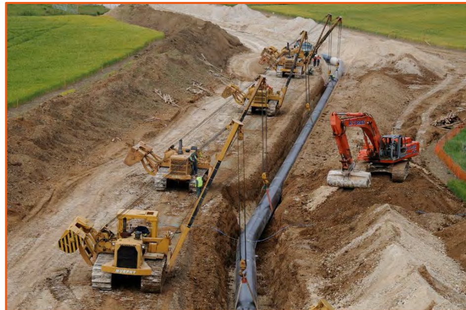
Trench opened and Pipeline lifted into position
