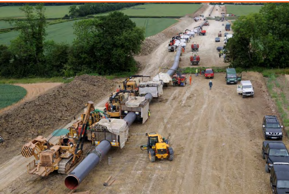
Pipeline welded in situ
