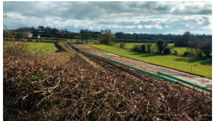
Welded pipeline ahead of ditching.
