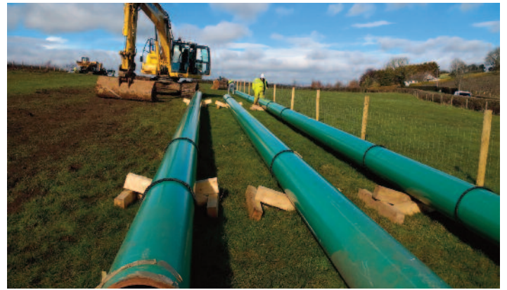
Pipeline stringing along the spread.
