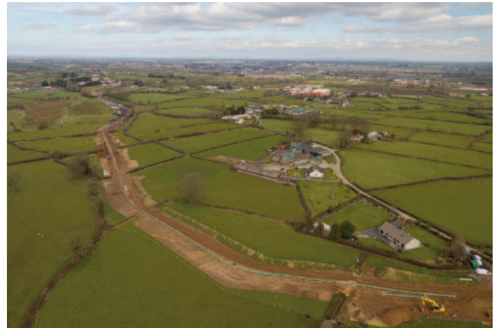
The pipeline between Coxhill Rd and the A3 South West of Portadown. This is an aerial view of the pipeline route showing welded pipe in advance of burial.
