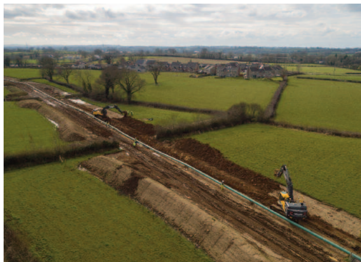
Pipeline being prepared for ditching close to Derryhale Road.
