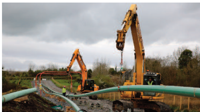
Pipeline being moved into position.
